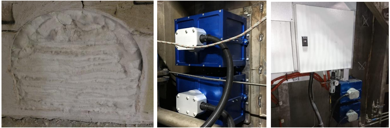
Figure 6. a) Installation of insulation fiber in front of sensor. b) Installed sensor housings at furnace. c) Radar central unit (DiRP) in apparatus housing with sensors.
